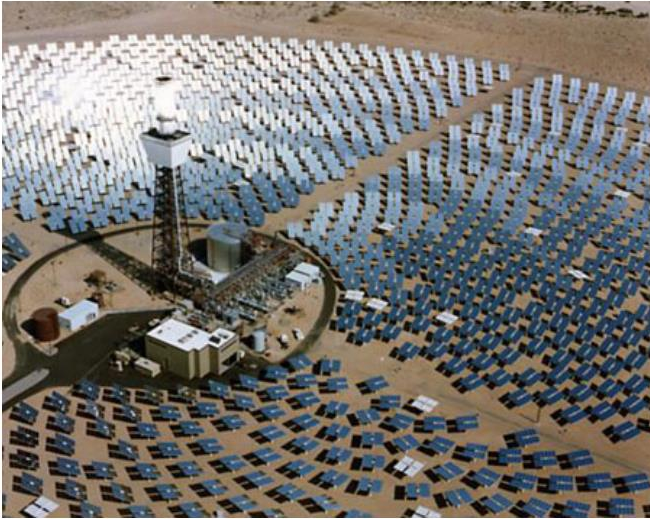
Solar Two - 81344m 2 collector. 48 MWth - 10.4 MWe
